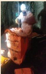
The material was loaded into the Hazibags and stored in the empty vaults. The Hazibags were then transported using sack trucks and loaded directly into a 35 yard container on a wait and load basis.
